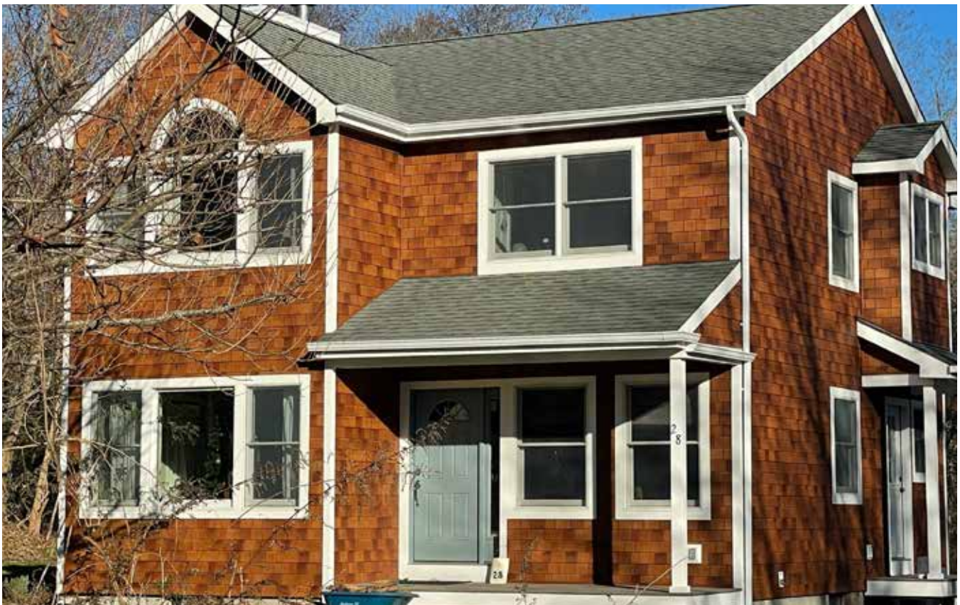
AFTER With Beach House Shake Pacifica Installed
